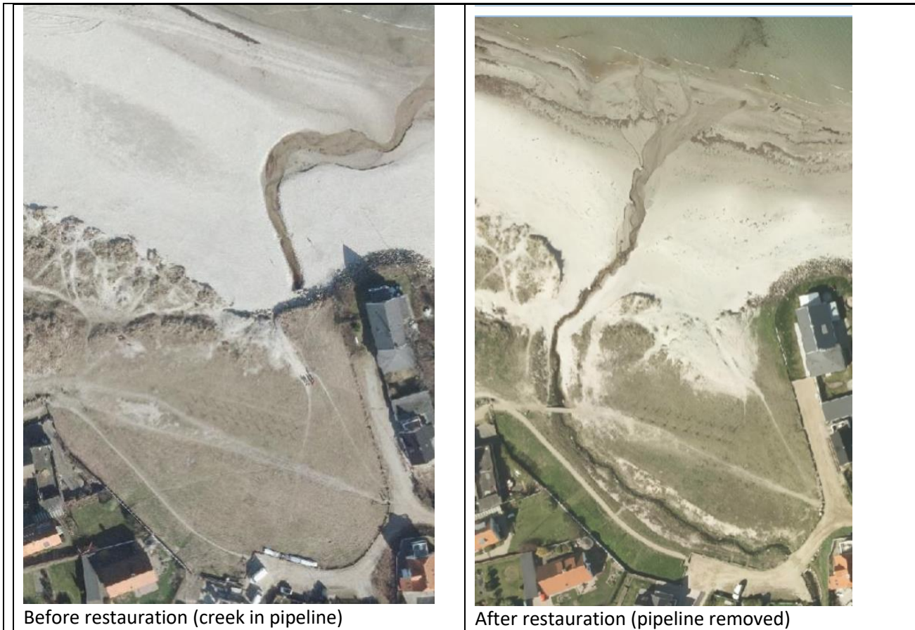
Figure 4.4. Oesterbaek in Hornbæk before and after restoration.
